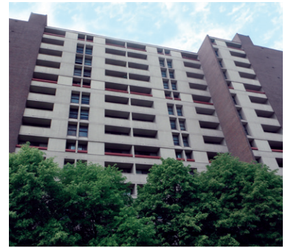
Bolton North apartment building
